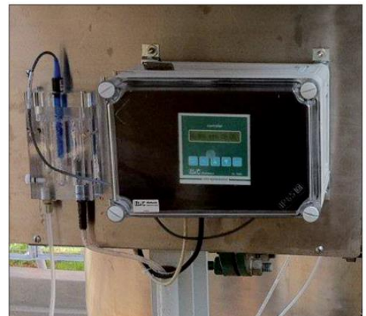
Typical installation example with controller CL7685 and flowcell SZ7231
